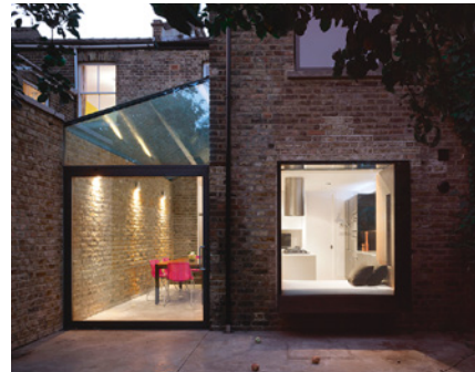
An angled glazing providing daylight to the extension without overshadowing the neighbor by Platform 5 Architects
